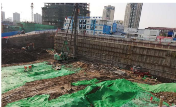
图 4 三轴搅拌桩施工图 Fig. 4 Sketch of construction of three-axis mixing piles
