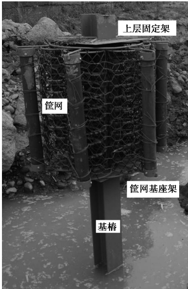
图 2 现地施做之筐网基桩 Fig. 2 Single pile with porous basket in field
