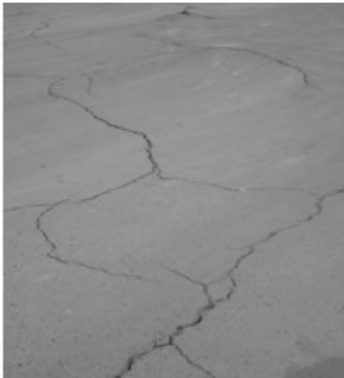
图 8 网裂并伴有凸起 Fig. 8 Mesh cracks with protruding
