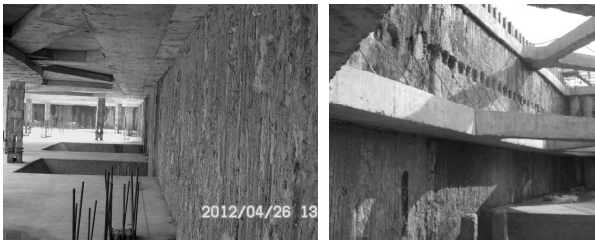
图 11 等厚度型钢水泥土搅拌墙侧壁实景 Fig. 11 Field picture of side wall
