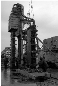
图 3 切割箱打入挖掘 Fig. 3 Cutting box being into ground
