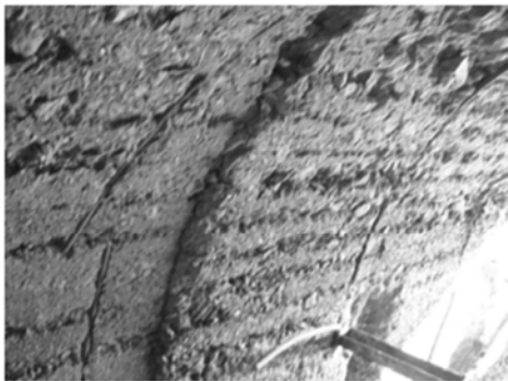
Fig. 9 Defects in the diversion hole
