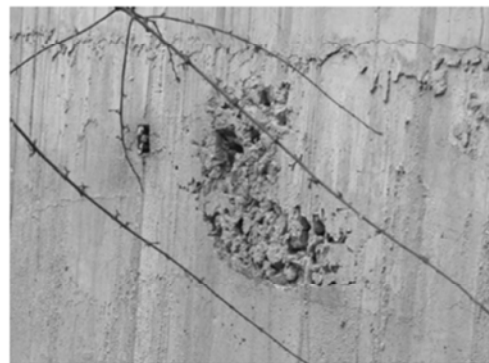
Fig. 6 Concrete spongy in right side
