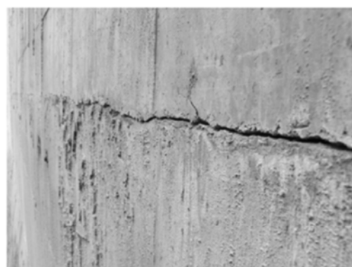
Fig. 2 Horizontal construction joints of upstream face
