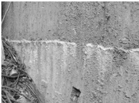
Fig. 7 Separation \text{CaCO}_3
