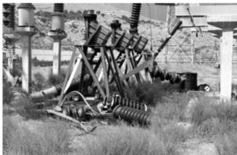
Fig. 5 Switchyard damage of Sefid Rud buttress dam caused by the 1990 Manjil earthquake, Iran
