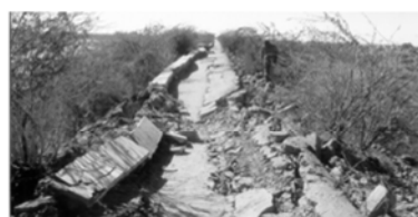
Fig. 1 Damage of concrete face of Zipingpu concrete face rockfill dam caused by the 2008 Wenchuan earthquake, China
