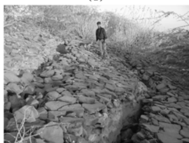
Fig. 2 Typical damage of embankment dams caused by the 2001 Bhuj earthquake, Gujarat, India
