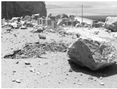
Fig. 4 Rockfall damage of Sefid Rud buttress dam caused by the 1990 Manjil earthquake, Iran
