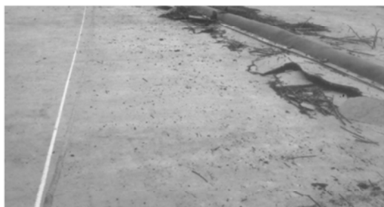
Fig. 1 Damage of concrete face of Zipingpu concrete face rockfill dam caused by the 2008 Wenchuan earthquake, China
