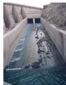
Fig. 3 Damage of Sefid Rud buttress dam caused by the 1990 Manjil (magnitude 7.5) earthquake, Iran
