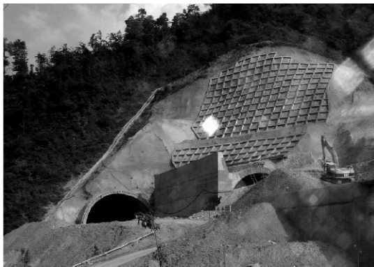
图 1 耳墙式隧道结构 Fig. 1 Tunnel structure with ear wall
