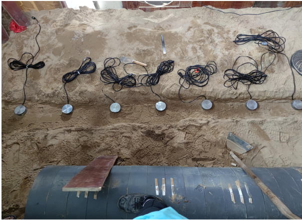
图 10 隧道底部土压力盒 Fig. 10 Earth pressure cells at tunnel bottom
