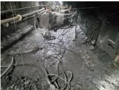
图 18 预制块反底拱现场施工图 Fig. 18 Construction drawing of precast block reverse bottom arch
