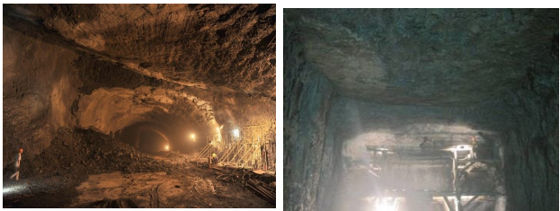
图 5 柱状节理玄武岩坍塌破坏 Fig. 5 Collapse failure of columnar jointed basalt
