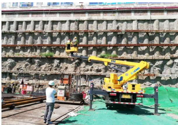
图 3 预应力锚索重新张拉施工图 Fig. 3 Sketch of re-tensioned locking of prestressed bolts
