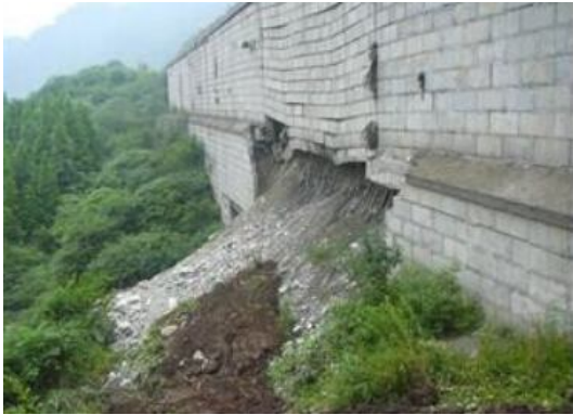
图 2 挡墙实际破坏情况 (西南交通大学研究组, 2009) Fig. 2 Actual failure of retaining wall (Study Group of Southwest Jiaotong University, 2009)
