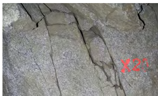
图10 PD24 洞深 0+88—0+89 m 上游壁的 N25°E 裂缝破裂特征 Fig. 10 Characteristics of N25°E orientation DSC at upstream wall of PD24 at depth of 88~89 m
