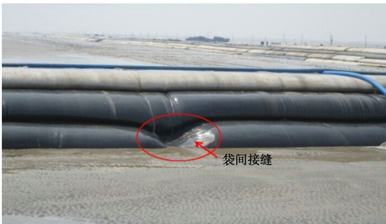
图 2 袋间接缝 Fig. 2 Seam between geotubes of geotube dam
