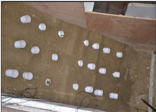
图 4 预留锚索施工孔 Fig. 4 Pre-reserved construction holes for anchor cables
