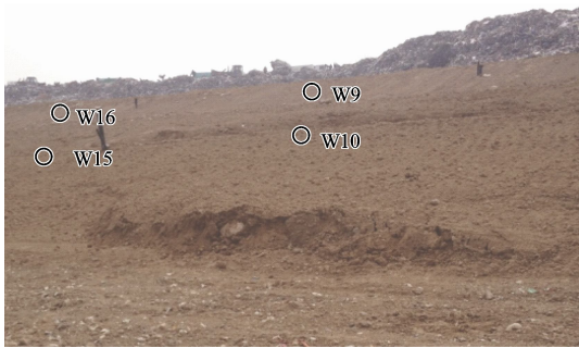
图 5 堆体边坡滑移形成的陡坎 Fig. 5 Scarp due to sliding of landfill slope
